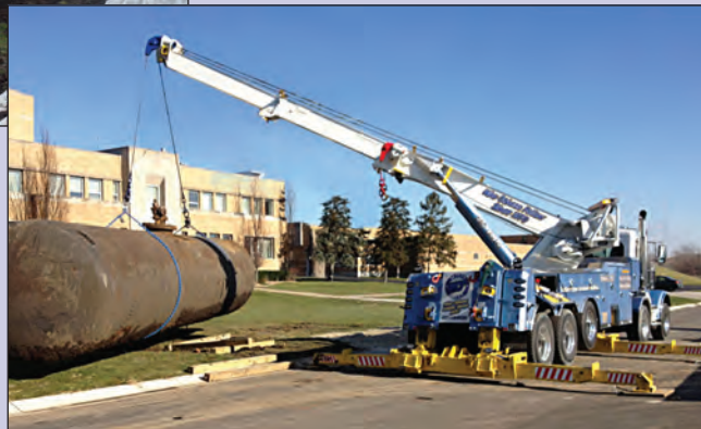
After removing the tank, it was loaded onto a waiting trailer for disposal.
