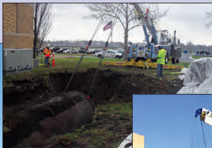
The tank was partially filled with water, making it a heavy lift.
