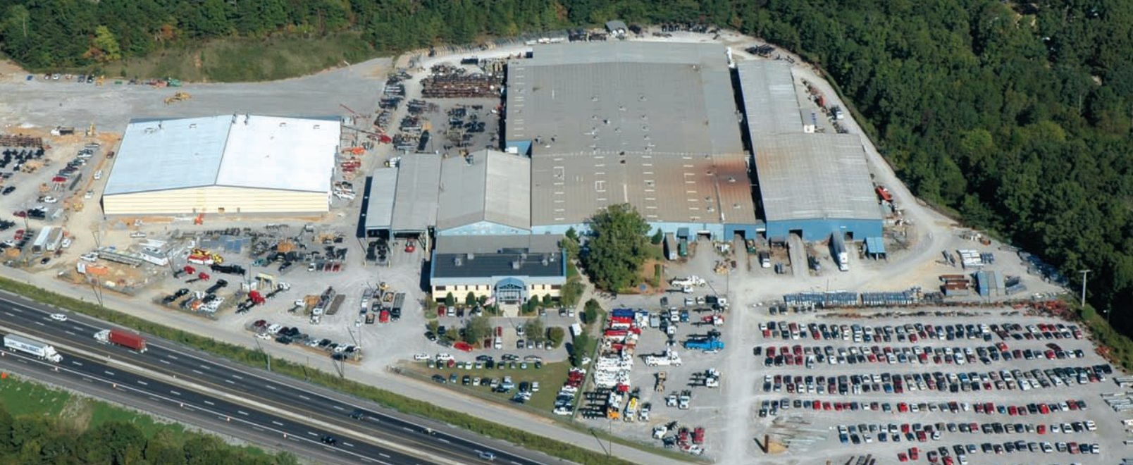
Miller Industries new 59,000 square foot, state-of-the-art light-duty manufacturing plant in Ooltewah, Tennessee, nears completion.
